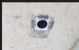
Metal boxes require extra plastering to cover mesh pattern
