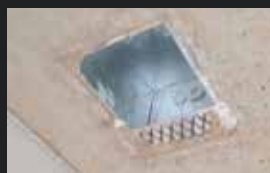
Metal boxes require extra plastering to cover mesh pattern
