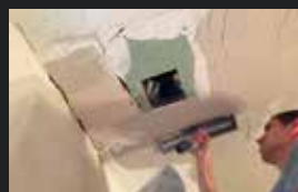
Metal boxes require extra plastering to cover mesh pattern
