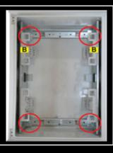
3) Fit the steel din rails (C), for breakers, into the plastic supports using 2 x 3.5 x 12 Panpozi thread cutter screws on each end as shown. Fit the steel din rail, for neutral bar, upside down using 2 x 8 x 9.5 thread cutter screws on each end as shown.
