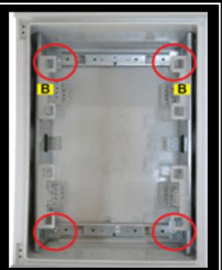
3) Fit the steel din rails (C), for breakers, into the plastic supports using 2 x 3.5 x 12 Panpozi thread cutter screws on each end as shown. Fit the steel din rail, for neutral bar, upside down using 2 x 8 x 9.5 thread cutter screws on each end as shown.
