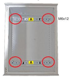
4) Fit the steel side plates with the plastic supports (B) onto the mounting rails (A) using the 4 x M6x12CH EG screws and M6 washers as shown.
